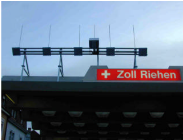
Figure 3-4: Multilane installation in Riehen
